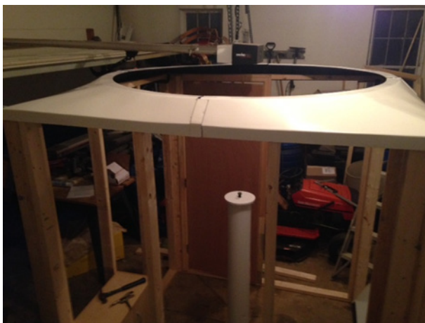
Figure 2: Construction of the telescope room for the MSRO. Source: Myron Wasiuta
