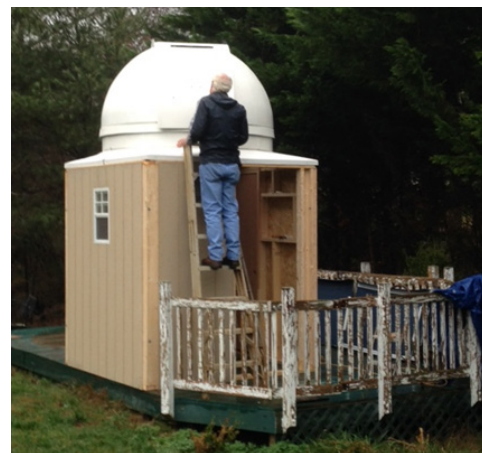
Figure 3: Ron Henke works on completing construction of the MSRO telescope room, including installation of the 6-foot Technical Innovations HomeDome. Source: Myron Wasiuta
